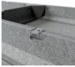
Box Tile Double Beams Clip Detail
