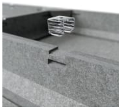
Box Tile Double Beams Clip Fixing Detail
